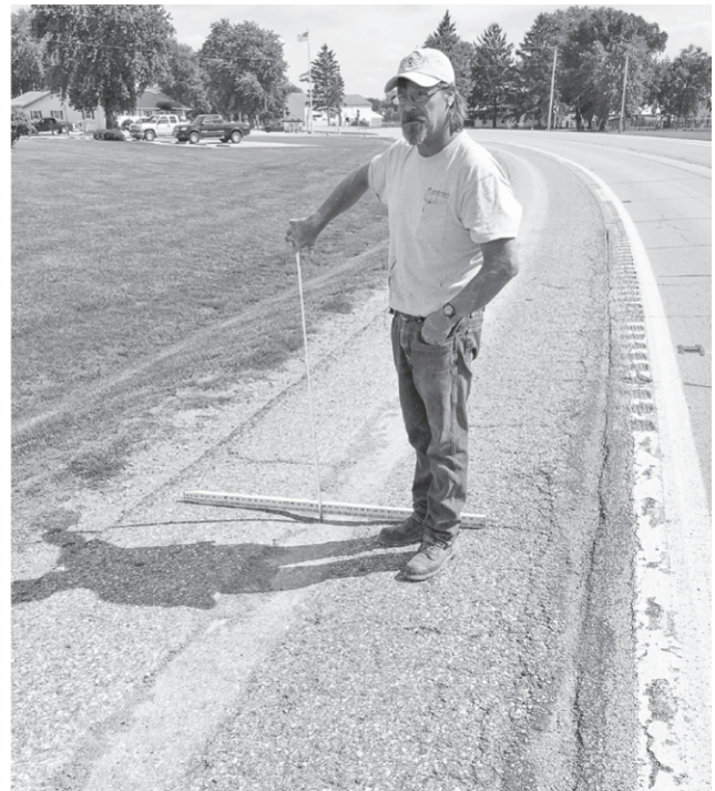
HIGHWAY COMMISSIONER Steve Helton shows the damage that horses have done wearing down roads in Bourbon Township (Douglas County).
